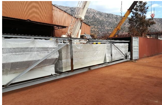
Figure 11. Unloading materials from a container.
