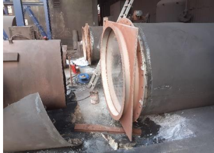
Figure 13. Flange welding at the tie-in.
